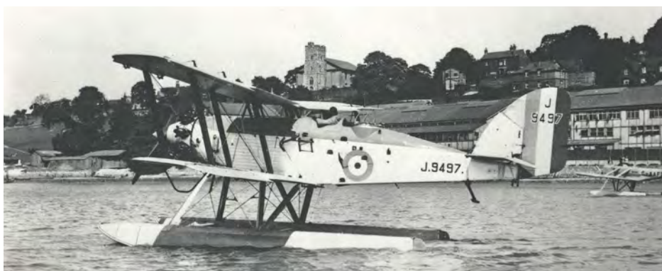
Below: The Wapiti was the most important design and manufacturing programme for Westland in the inter-war period. It could be configured as a landplane or with floats, like this Wapiti IIA seaplane, J9497.
