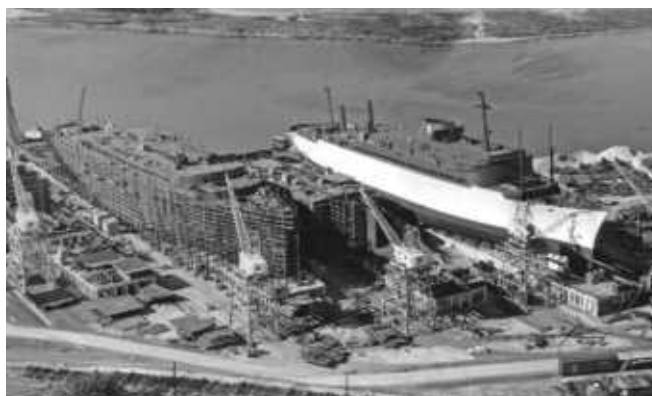
▲ Built simultaneously and with prefabrication, the twins had their familiar look as Brasil (right) is prepared for launch in December 1957.
