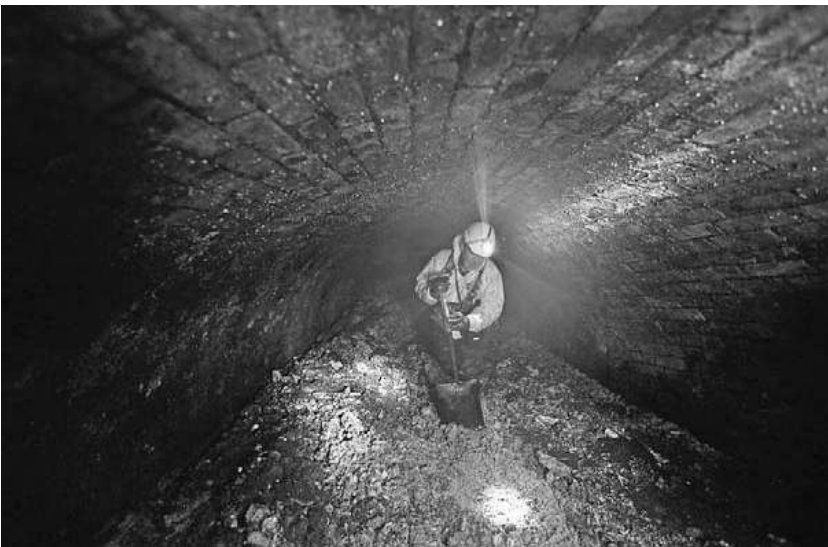
Working in the London sewer in 2014. A fatberg — an agglomeration of fat, disposable wipes, diapers, condoms and tampons — found in the sewer weighs more than 140 tons.
