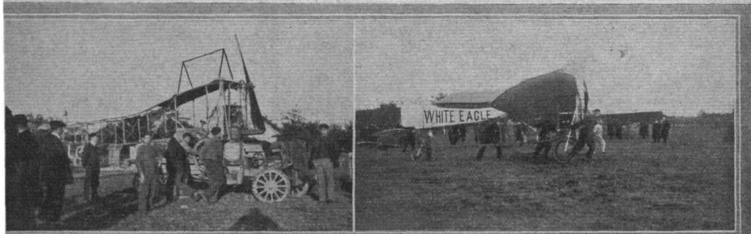
AT PAU.—On the left, arrival of Mr. Claude Grahame White's two-seated, type XII, Bleriot monoplane, fitted with a 60-80-h.p. E.N.V. engine, at Pau Aerodrome on November 24th last. On the right, starting for a trial run on November 28th, on Mr. Grahame White's "White Eagle." On this occasion an officially-timed circular flight of 6 kiloms., at a record speed of 96 k.p.h., with a passenger up, was made.
