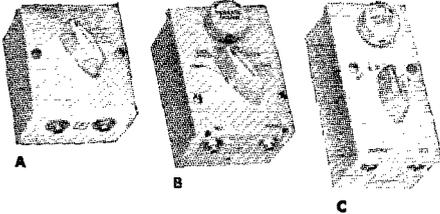
(A) BC-345, 3 1/2" x 3" x 1 7/8" aluminum, 2 standard open-circuit jacks, 3-position switch, 6-contact banana plugs and jacks.
