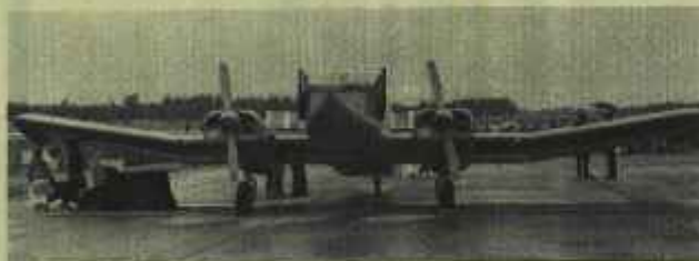
The simple construction of the Evangel 4500 is evident in the square fuselage section and straightforward Jodel-style cranked wing. The use of 2024-T3 Al. aluminum skinning is claimed to make field repair easier. See story on this page
