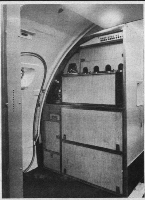
A typical aircraft galley installation, designed and built by Henshall's of Byfleet for the H.S.A. 121 series 1.E A/C. This unit incorporates universally used heated Beverage Containers, Food Ovens, Meal Tray Boxes, Bar Boxes, etc., all made by Henshall's, who are suppliers to the leading British and foreign airlines.
