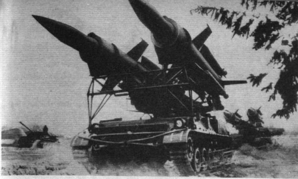
These four pictures were recently issued from Russia. Though showing the customary retouching and fogging, they offer a rare glimpse of Russian missiles in operation. Above are two pairs of the ramjet propelled surface-to-air missiles first seen last May
