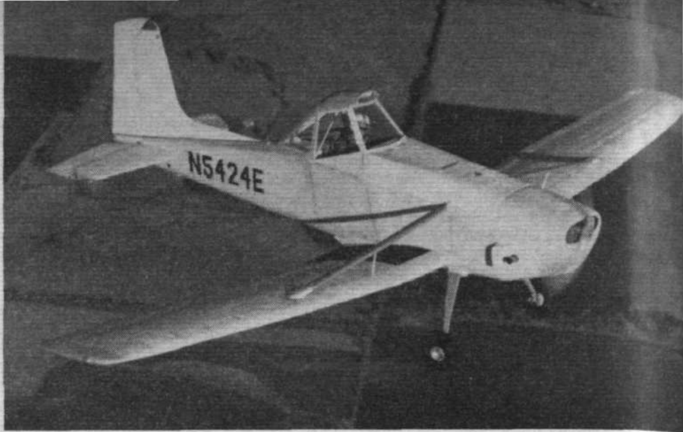
On February 19 Cessna flew a new single-engined agricultural aircraft called the Agwagon. Production plans will not be completed until the prototype has been tested under actual operating conditions. Meanwhile details are being withheld, but the aircraft clearly uses many Skywagon components
