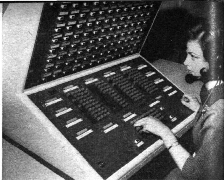
Keyboard for the Elliott 100-track radar target simulator
