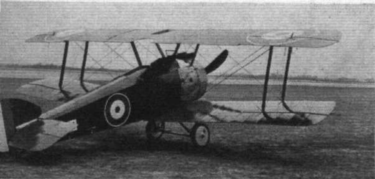
RESTORED to flying trim by Mr. Frank G. Tallman, of Chicago, is this Sopwith Camel F.1, with 110 h.p. Le Rhône engine. Except for steel undercarriage struts, the machine is considered to be accurate in every detail.
