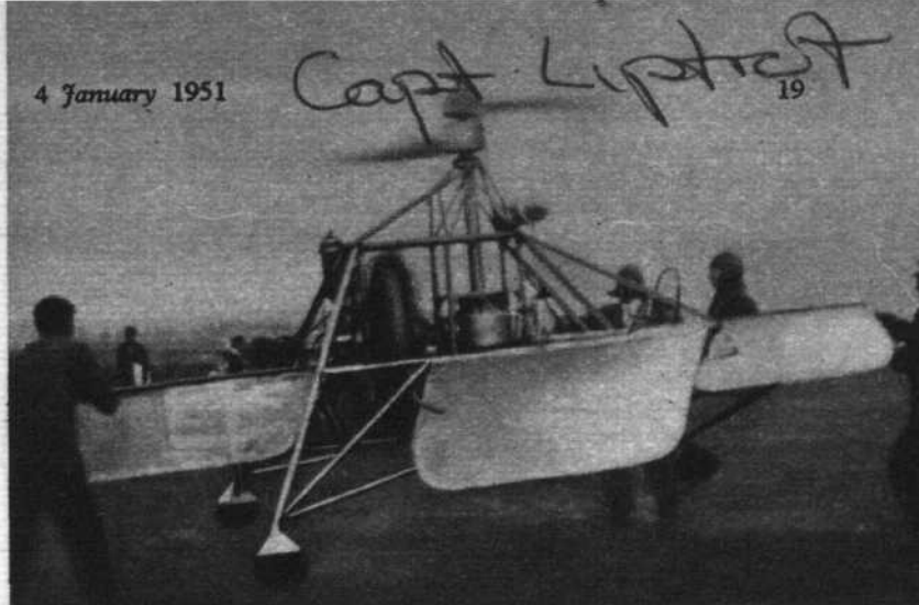
Asboth's fourth helicopter (1930). The machine is seen coming in to land, with the author at the controls.
