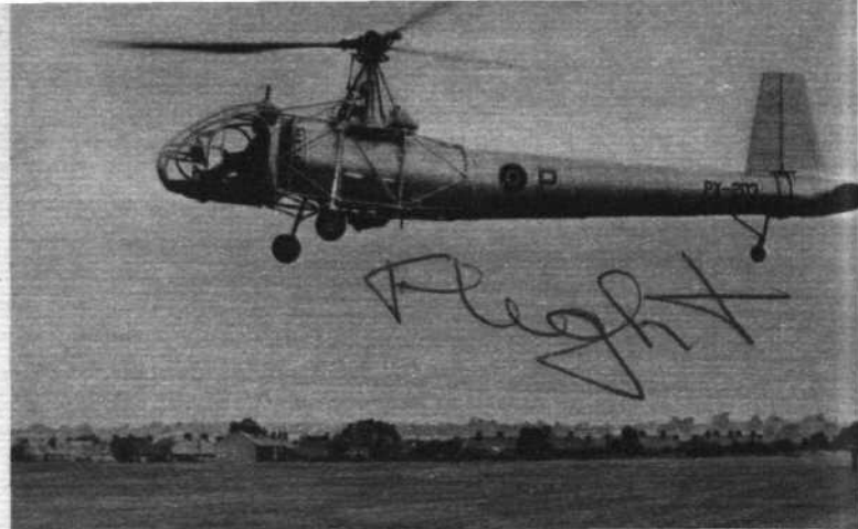
Cierva W.9, with jet reaction at the tail for torque compensation.
