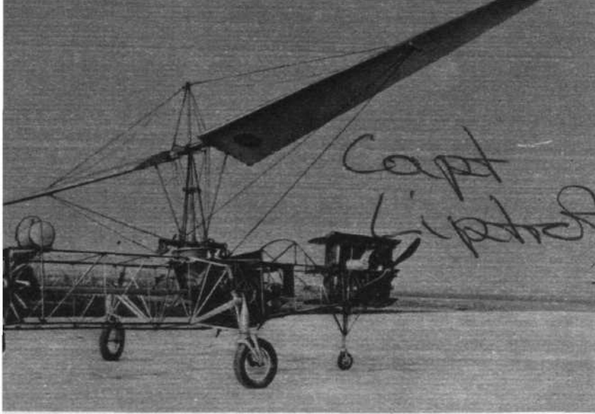
Von Baumhauer helicopter of 1924—first with single main rotor and tail torque-compensating airscrew. Forerunner of classical Sikorsky types.
