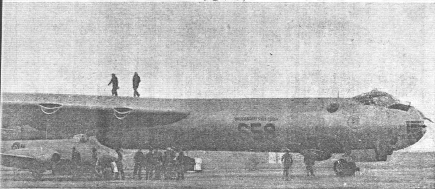
A Gloster Meteor 4 acts as a yardstick for one of the visiting B-36s. Respective lengths of the two machines are 43ft 6in and 162ft. The B-36 depicted has yellow nacelle-noses and nosewheel doors, yellow-tipped vertical tail surfaces, brown and green radar blister, and black identity markings. Emblazoned on the fin is the insignia of the 8th Air Force. All barbettes are retracted and quite invisible. Armament is sixteen 20 mm guns.
