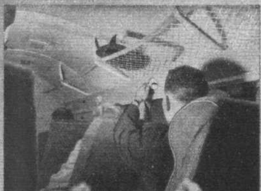
VENTILATION: There are eight individually adjustable cold-air louvers. Hot-air ventilation is controlled by the crew.
