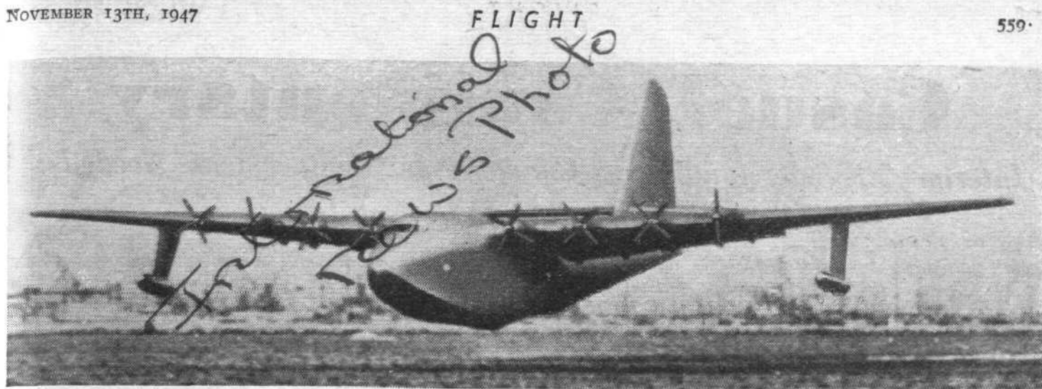
SARGANTUAN GRACE: Despite its vast size (the span is 320 ft) the Hughes Hercules, seen airborne, with Mr. Howard Hughes at the controls during taxiing tests on November 2nd, has fine lines. The eight Wasp Majors deliver an aggregate of 24,000 h.p.
