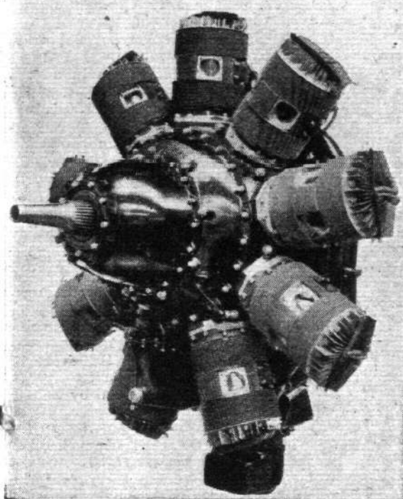
Bristol's first sleeve-valve research started in 1927 and resulted in the 580 h.p. Perseus of 1932.
