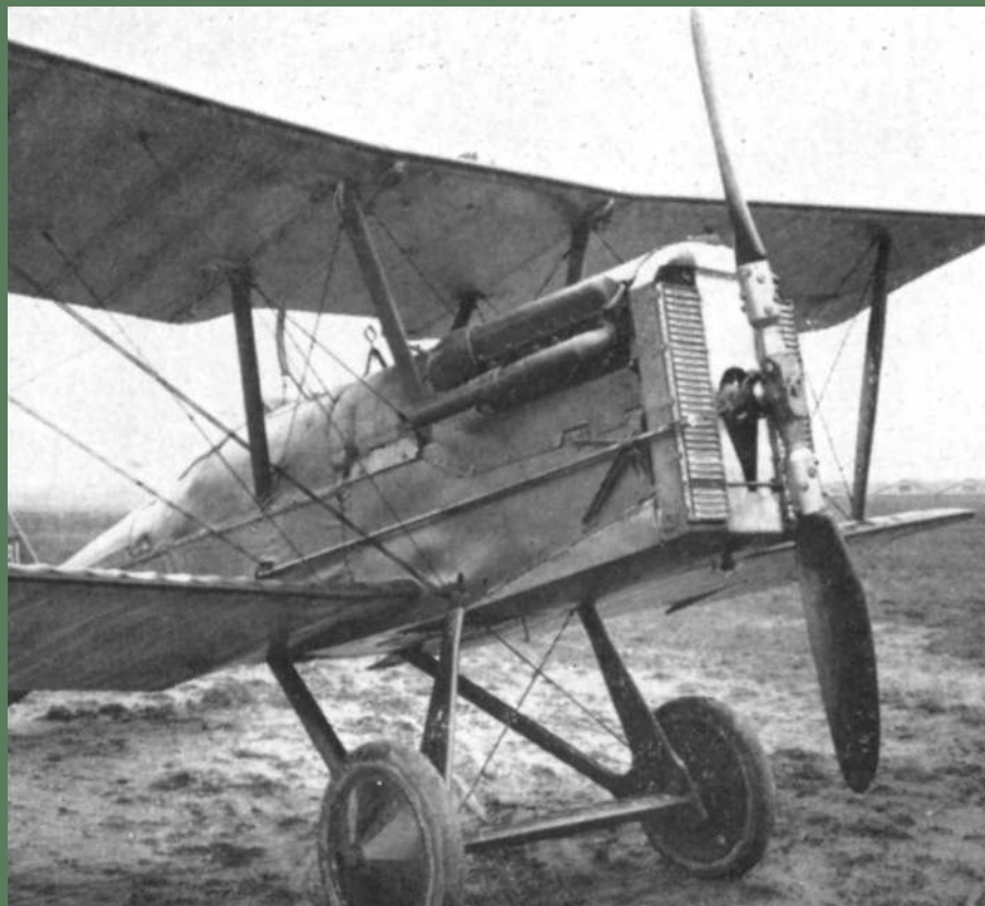
A post WW-1 experiment applied to this S.E.5a was this variable pitch propeller, undertaken during 1920.
