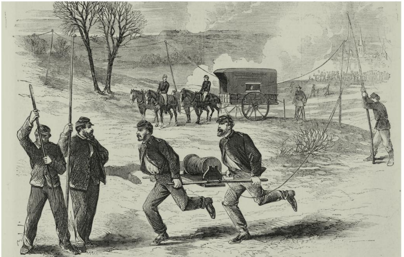
LINES OF COMMUNICATION Troops lay telegraph wire at Fredericksburg, Virginia. Tapping of telegraph lines was rampant, making Confederate general Robert E Lee distrustful of the medium because of the ease with which messages could be intercepted
